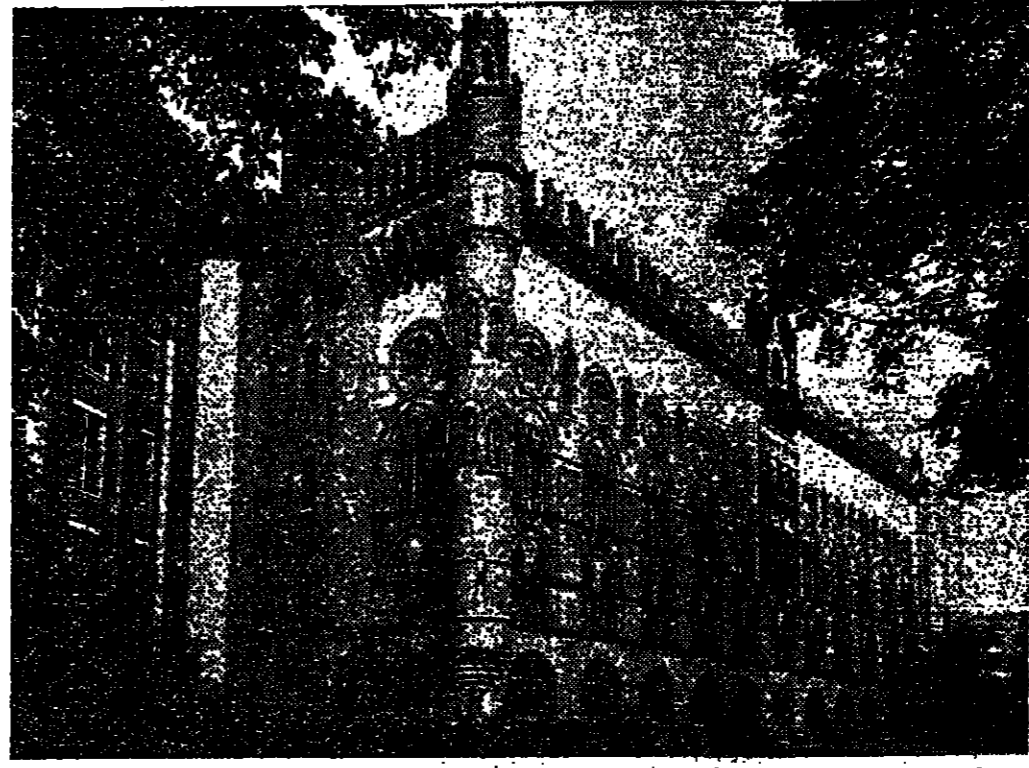
One of Glasgow's most famous factory buildings, known as the "Doges Palace," part of a complex totalling 385,000 square feet on a four-acre site, is to be sold by the British Carpets subsidiary of Guthrie Corporation.
